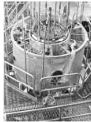
Fig. 1. STEK facility - Top View
