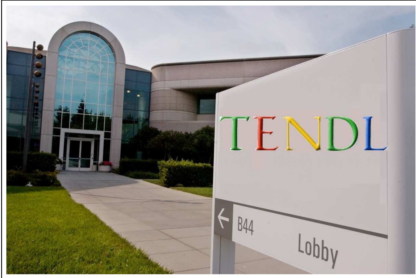
The TENDL building (2014)
